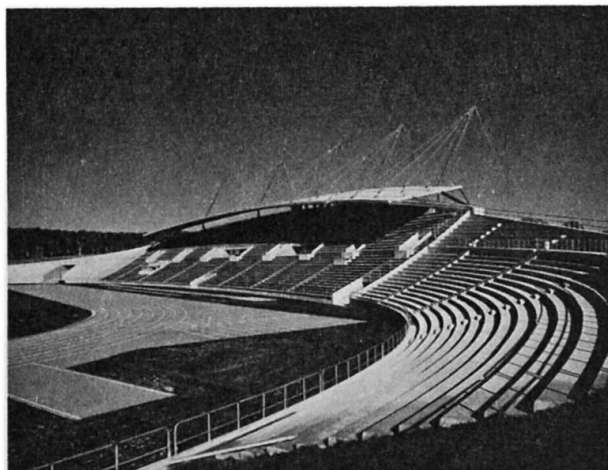
View from inside the stadium showing the grandstand with its cable suspended roof.
