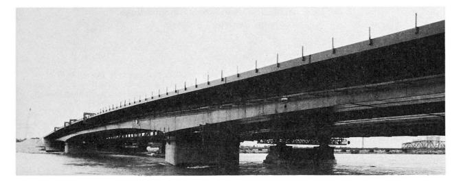
A grillage comprising 40 drilled piles, each 17 m long with a diameter of 1.2 m, was made for the river piers. At river bed level the piles were joined by means of a reinforced concrete slab. An apron made of sheet pile wall planks was sunk down to a depth of 8.5 m to counteract floodwater pit formation and erosion. The reinforced concrete river pier was built upon this base structure and protected against erosion from sediment transport by a specially wear-resistant facing layer.
