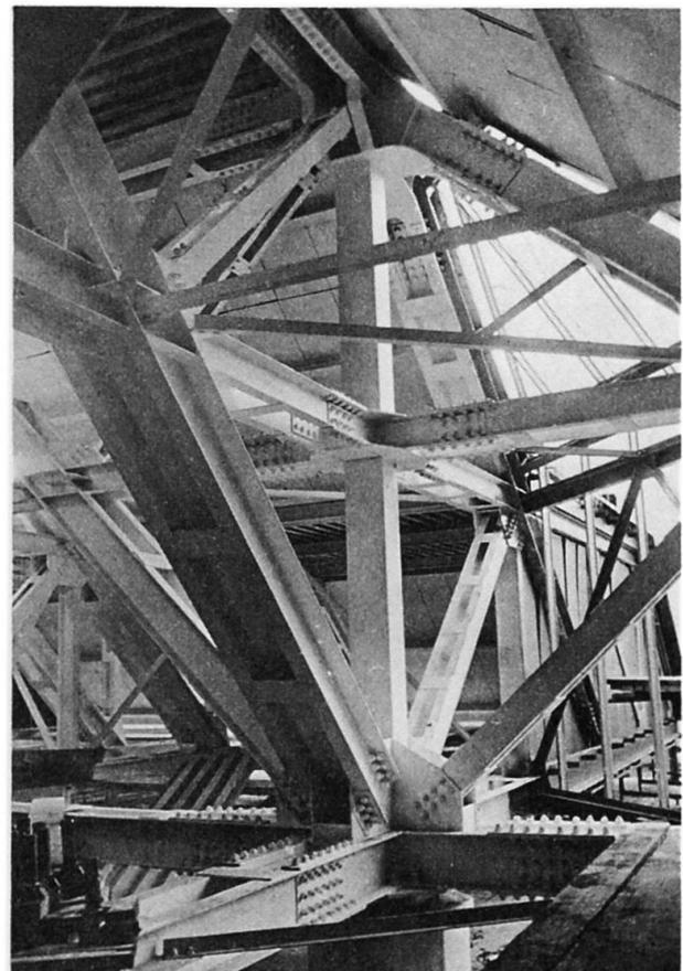
This structure arranged around the center building is self-supporting and not connected to the center building. The construction is of bolted design.
