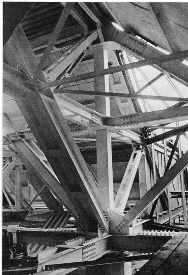
This structure arranged around the center building is self-supporting and not connected to the center building. The construction is of bolted design.
