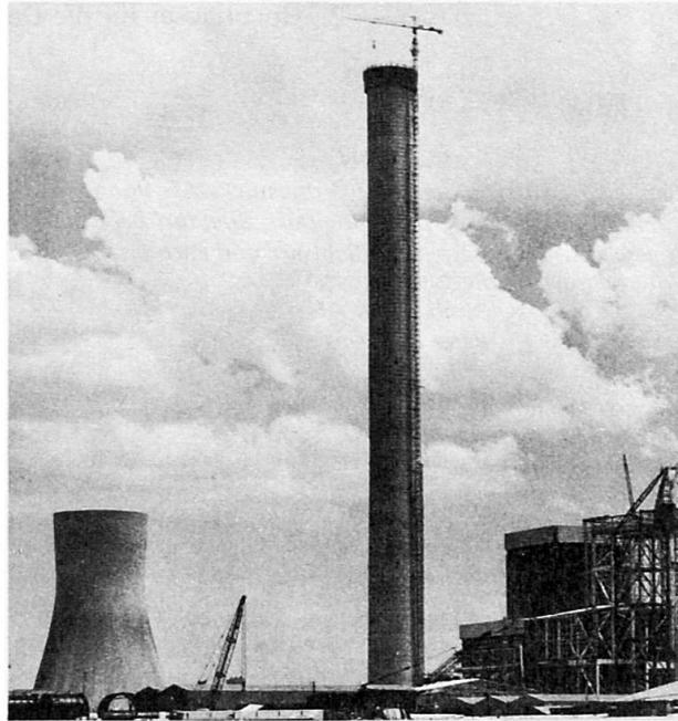
Generally the flue lining is a single 110 mm thick brick skin although in certain areas, for example at the flue inlet, a double brick skin of 230 mm thickness is used.
