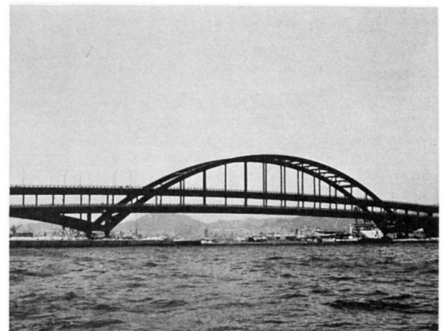
KOBE OHASHI BRIDGE (KOBE CITY)
