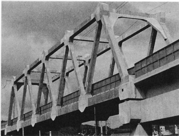
Photo 3 Prestressed concrete truss bridge
