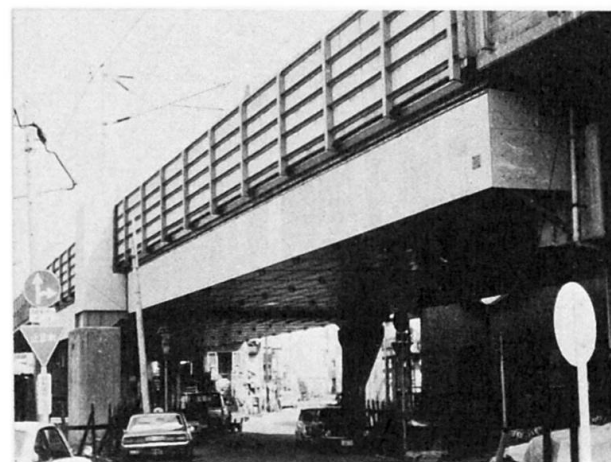
Photo 2 Bridge after improvement
