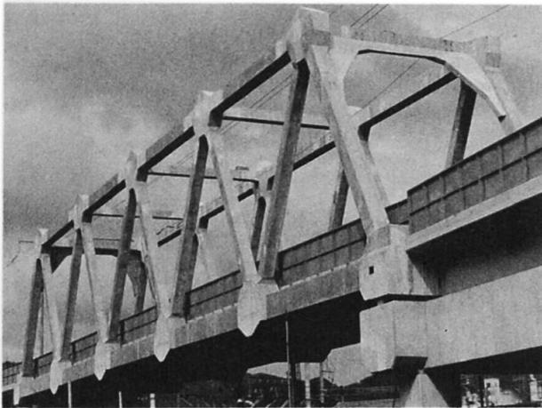
Photo 3 Prestressed concrete truss bridge
