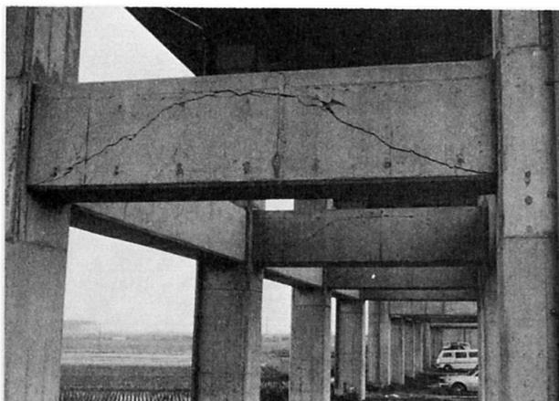
Photo 1 Damage in beam of concrete viaduct
