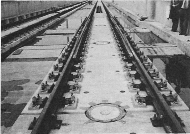
Photo 3 Expansion rail joint for slab type track
