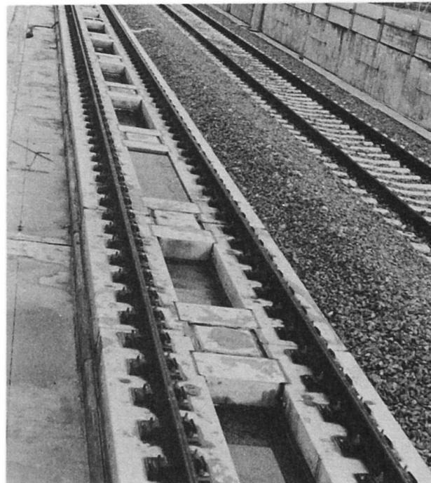
Photo 5 Anti-vibration slab track with precast concrete frames
