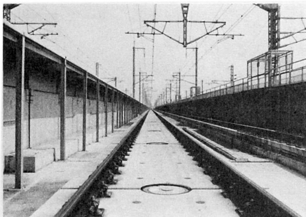
Photo 1 Slab type track
