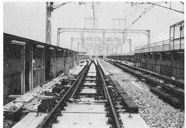
Photo 2 Turnout for slab type track
