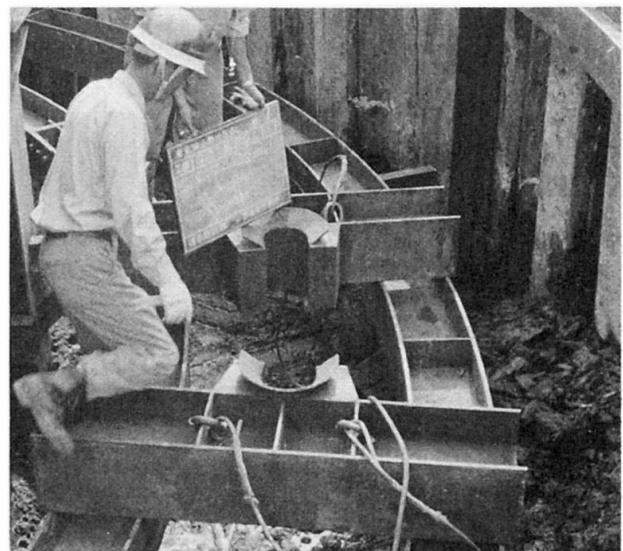
Photo 2 Guiding ring beams for pipe-pile-wall foundation
