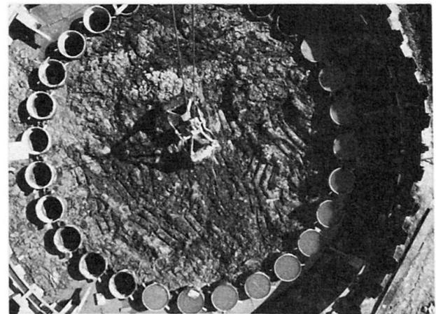
Photo 1 Circular arrangement of pipe-pile-wall
