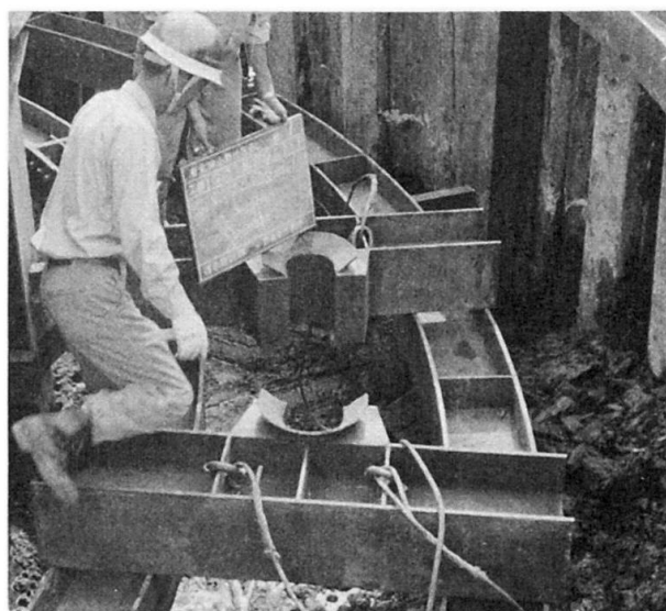
Photo 2 Guiding ring beams for pipe-pile-wall foundation
