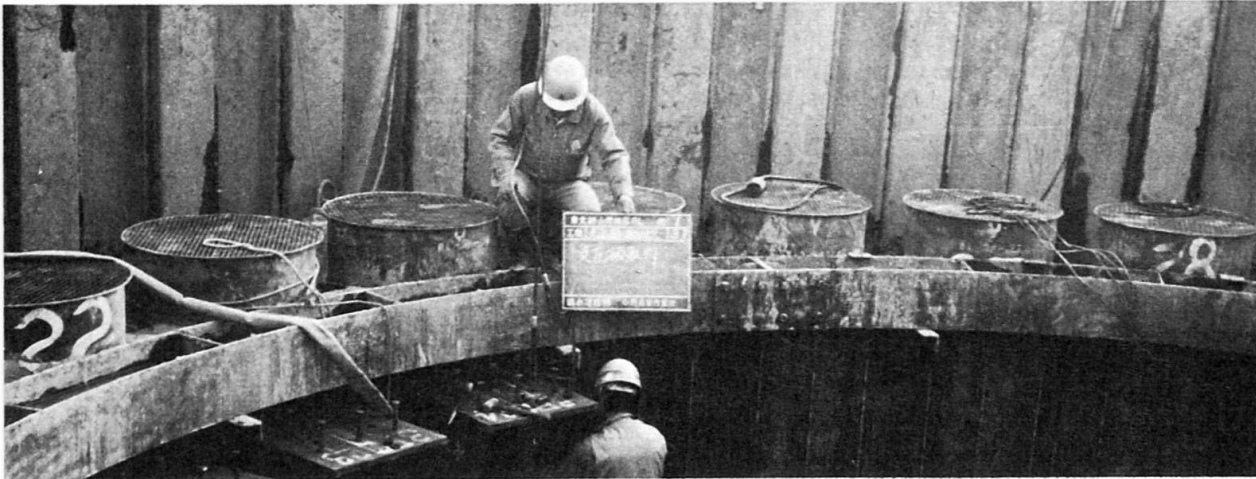
Photo 3 Brackets to support top slab
