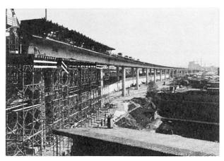
The load bearing subsoil strata of Rhein gravel lies at varying depths up to 10 m below ground level and is overlain by a strata with a very poor bearing capacity. Pad or piles foundations were used, depending on the depth at which the gravel was found. In case of piling, bored piles with a dia. of 116 cm were chosen.
