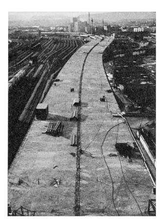
This 1,5 km long bridge connects the Swiss National Motorway N2 with the German Hafraba Motorway, linking Hamburg with Basle (E4). Starting at the joint customs facilities located on German territory, the bridge crosses the territorial boundary, following the embankment of the German Federal Railway (DB) until it reaches the large, common abutment of the bridge over the river Wiesen.
