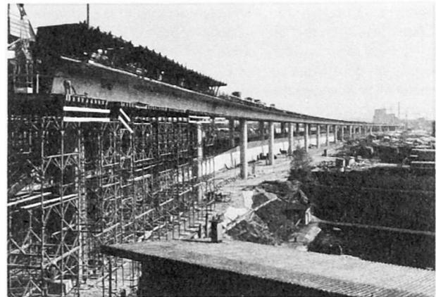
The load bearing subsoil strata of Rhein gravel lies at varying depths up to 10 m below ground level and is overlain by a strata with a very poor bearing capacity. Pad or piles foundations were used, depending on the depth at which the gravel was found. In case of piling, bored piles with a dia. of 116 cm were chosen.
