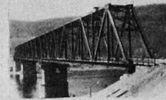
Steel Railway Bridge on the Baikal - Amour Railway Line Steel continuous girder with spans 110 + 132 + 110 m
