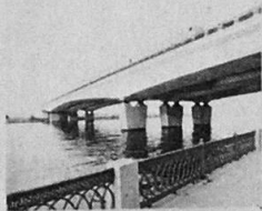
Bridge over the River Moscow Concrete continuous girder with spans 62 + 114 + 62 m (for combined traffic of city vehicles and Metro trains)
