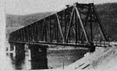
Steel Railway Bridge on the Baikal - Amour Railway Line Steel continuous girder with spans 110 + 132 + 110 m
