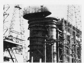
Fig. 2 Erection of Stoves
