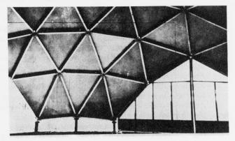
Fig. 3 Interior View of the Latticed Spherical Shell
