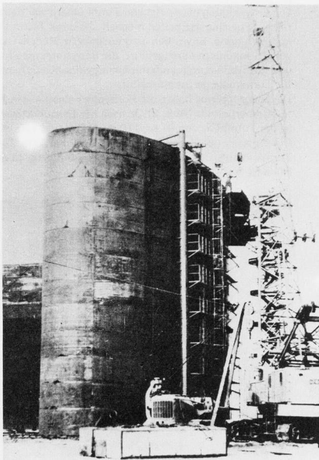
Fig. 2 Erection made by a Roll Forming Method
