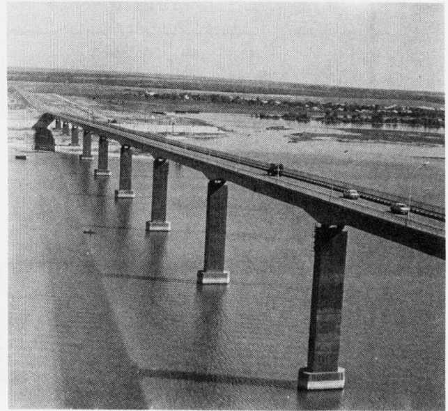
Fig. 1 The general view of the bridge
