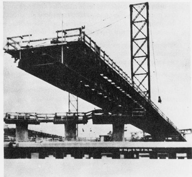
Fig. 4 Erection of the superstructure steel unit by longitudinal launching
