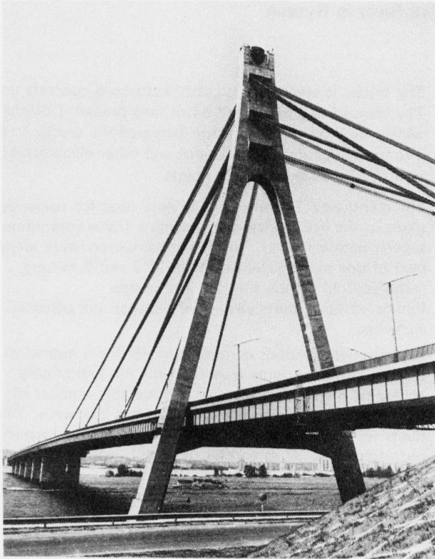
Fig. 5 General view of the bridge over the river Dnjepr in Kiev
