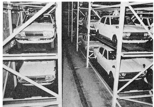
Automated warehouse (Nissan Motor Co., Ltd.)
