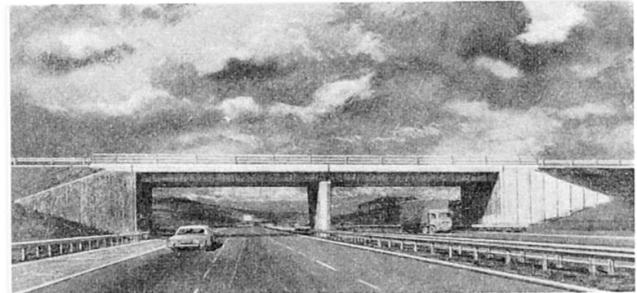
Fig 6 a 2 span overbridge of U beam construction
