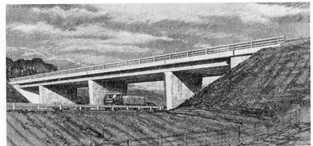
Fig 7 a 4 span overbridge of M beam construction
