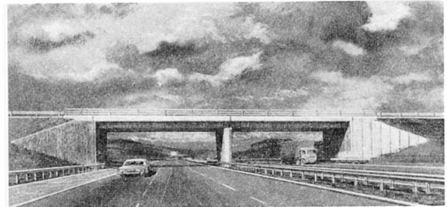
Fig 6 a 2 span overbridge of U beam construction
