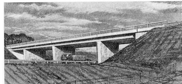
Fig 7 a 4 span overbridge of M beam construction
