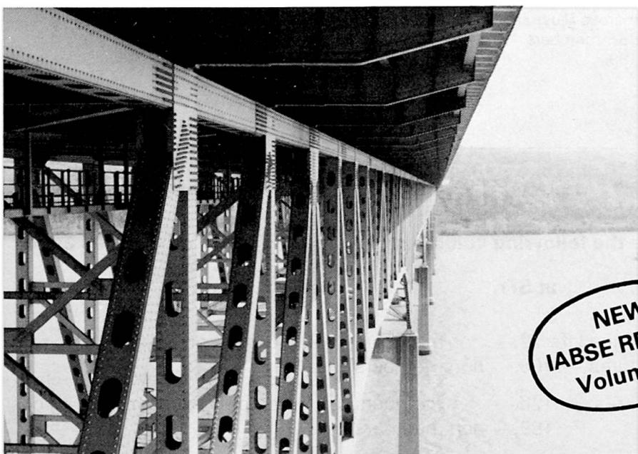
Fig. 12 Truss System of the Susquehanna River Bridge
