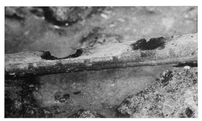
Localised corrosion on steel in concrete
