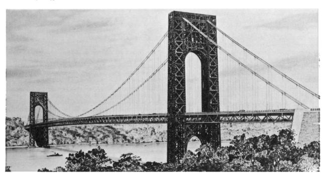
George Washington Bridge, New York, built 1927 - 1931; Construction underdeck 1962; Span 1067 m
