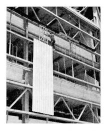
Fig. 33. Erection of wall panel.
