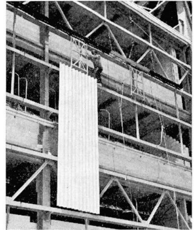
Fig. 33. Erection of wall panel.
