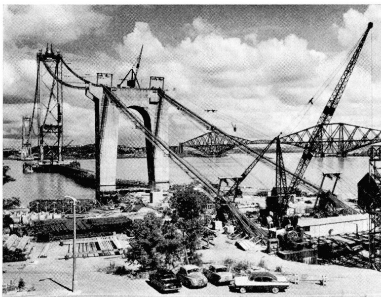
Fig. 6. A general view taken on last day of cable spinning.
