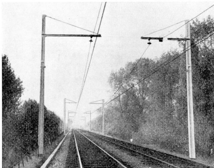
Fig. 1. Prestressed Concrete Cantilever Masts near Southend (England).
