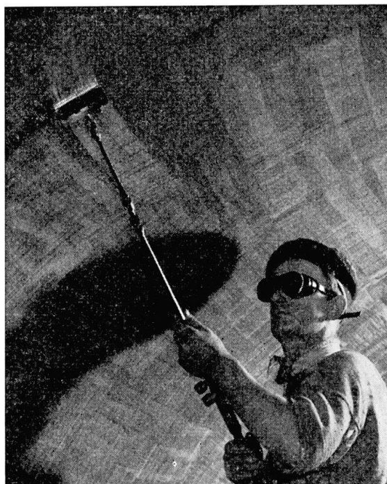
Fig. 12. Flame-cleaning in operation.
