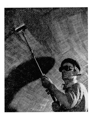
Fig. 12. Flame-cleaning in operation.
