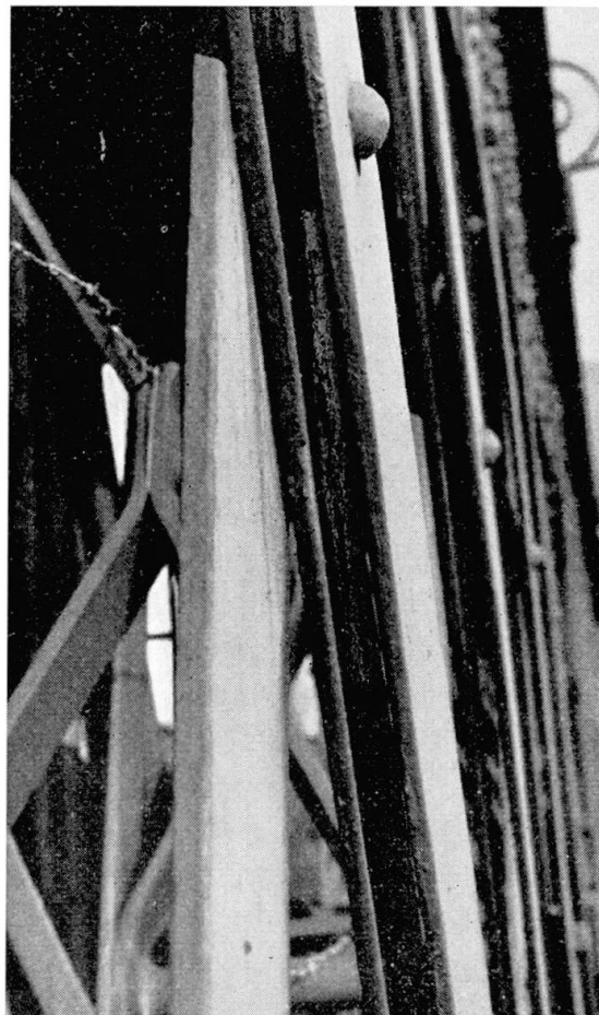
Fig. 9. Influence of design on corrosion. Difficult access to surfaces for repainting (railway bridge at Putney).
