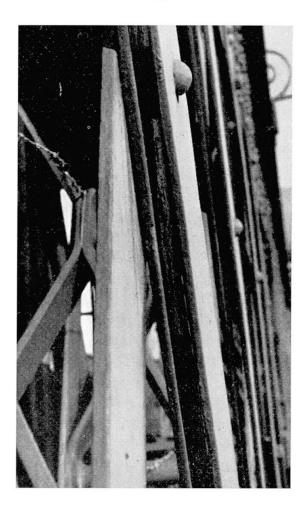
Fig. 9. Influence of design on corrosion. Difficult access to surfaces for repainting (railway bridge at Putney).
