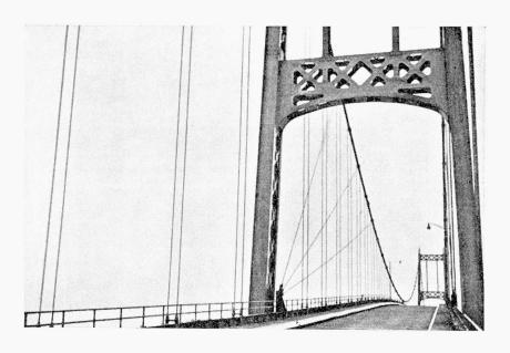
Fig. 24. Cable Stays for Checking Aerodynamic Oscillations. Installation on Thousand Islands Bridge and Deer Isle Bridge, 1938.
