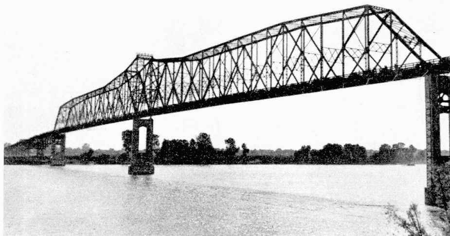
Fig. 3. Continuous Truss Bridge over the Mississippi River at Chester, Illinois. Destroyed by Wind, July 29, 1944.
