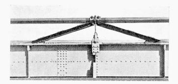
Fig. 23. Mid-Span Stays for Preventing Torsional Oscillations. Installation on Thousand Islands Bridge and Deer Isle Bridge, 1938.
