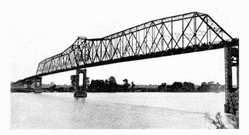
Fig. 3. Continuous Truss Bridge over the Mississippi River at Chester, Illinois. Destroyed by Wind, July 29, 1944.
