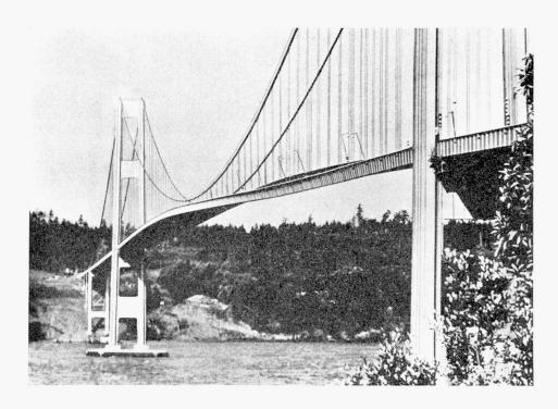
Fig. 1. Catastrophic Aerodynamic Oscillations of the Tacoma Narrows Bridge. Torsional Oscillations, November 7, 1940. Maximum Double Amplitude, 28 feet.
