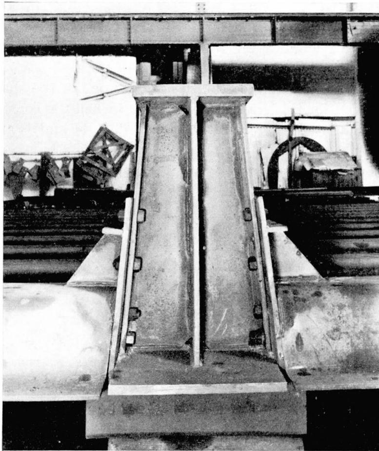
Fig. 12. The bridge shown in fig. 11. Details of the bolted connections of the ballast plates to an intermediate main girder
