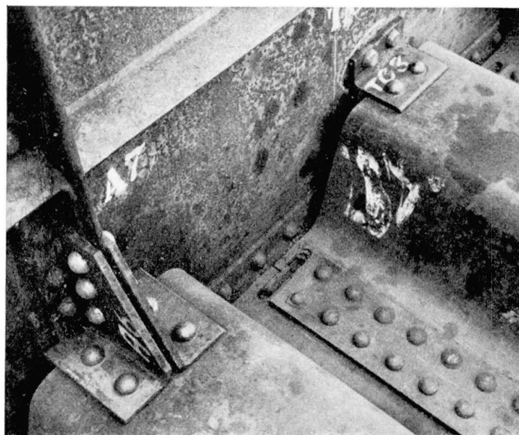
Fig. 13. Transverse pressed steel troughing connected to a main girder by cleats at the top and by plug-welds at the bottom
