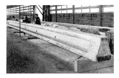
Fig. 5. Checking test bridge beam 50 ft. at Shorne 1952
