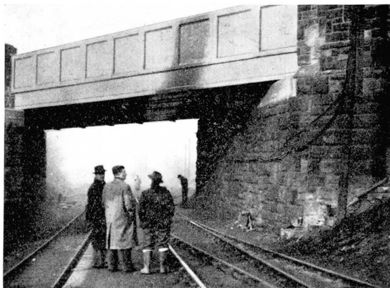
Fig. 7. Silverwood bridge, completed structure 1952
