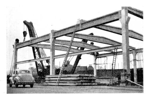
Fig. 11. Bury St. Edmunds. Prestressed beams of first part of roof
