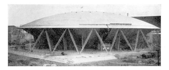
Fig. 2. Dome complete except for Apron Sheets, 28/10/50
