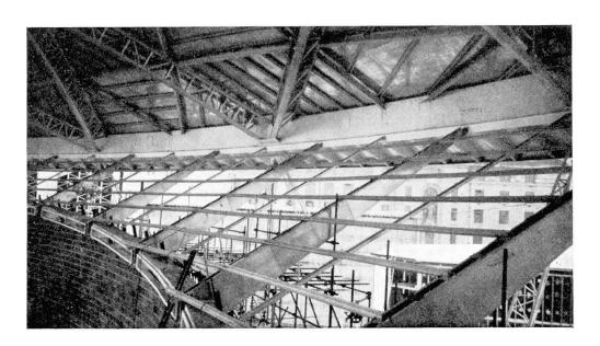
Fig. 15. Details of connections to Ring Girder, 26/9/50
