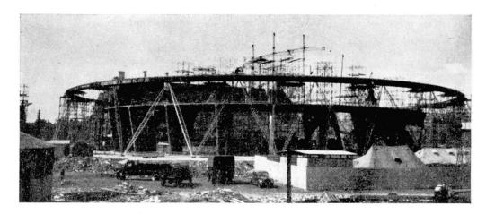
Fig. 9. Ring Girder and Struts complete. First arch being erected, 15/6/50
