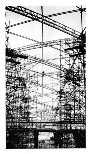
Fig. 10. Aligning rafters. *Note* main rib on left, 24/8/50
