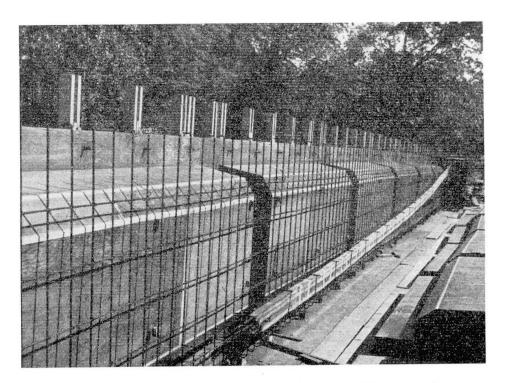
Fig. 4. Formwork Details, Reinforcing Steel and Rubber Cores
