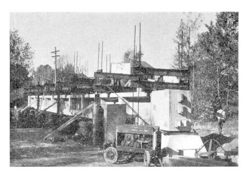
Fig. 12. View of Test Girder and Loading Arrangement Looking northwest, after loading up to 3000 lbs. per foot. Instrument shelter in the foreground
