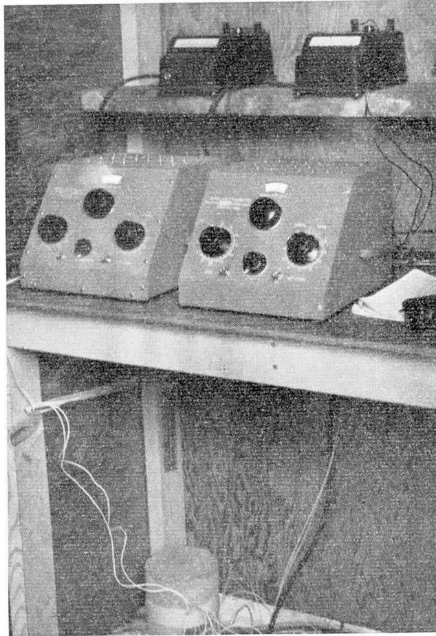
Fig. 11. Strainmeters and Compensator Gage
