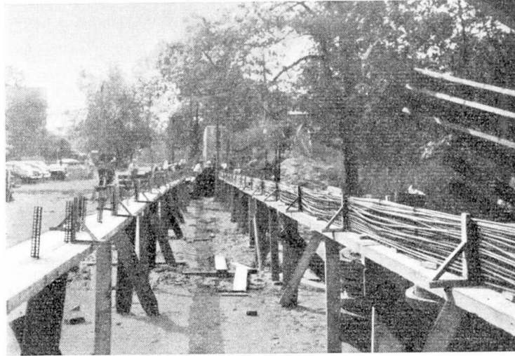
Fig. 5. Cable Assembly and Comb Spacers
