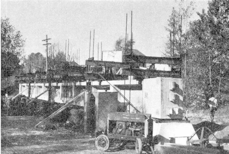
Fig. 12. View of Test Girder and Loading Arrangement
