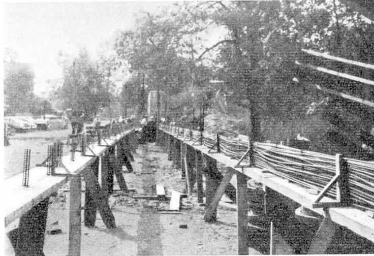
Fig. 5. Cable Assembly and Comb Spacers
