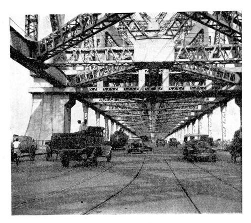
Fig. 5. Suspended deck viewed through main tower.
