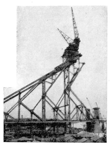
Fig. 4. Erection of Howrah Anchor Arm nearly completed.
