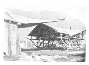
Fig. 29. Coffrage. — Schalung. — Forms and false-work.
