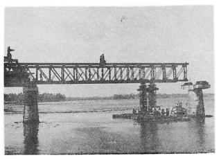
Fig. 4 Movement of Assembly Truss
