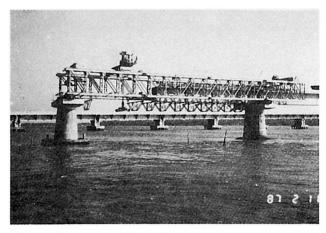
Fig. 3 Assembly of Segment
