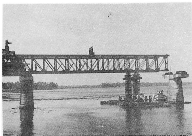
Fig. 4 Movement of Assembly Truss
