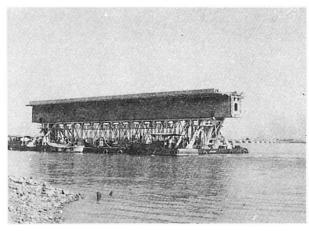
Fig.2 Girder being transported on a pontoon
