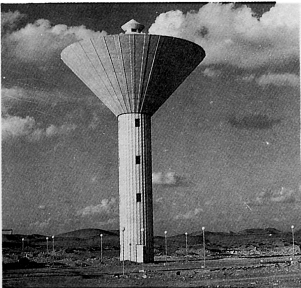
Fig.33 Haza Al Maqam reservoir, U.A.E.
