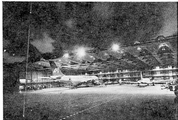
Fig.21 Indian Airlines Hangar, Bombay
