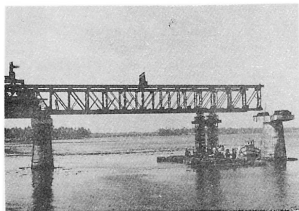
Fig. 4 Movement of Assembly Truss
