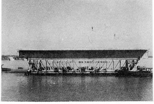
Fig. 4 Girder being towed to location
