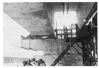
Fig. 5 Girder about to be placed
