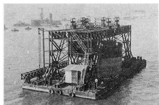
Fig.7 Cofferdam being lowered
