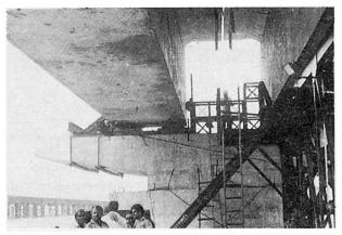
Fig. 5 Girder about to be placed
