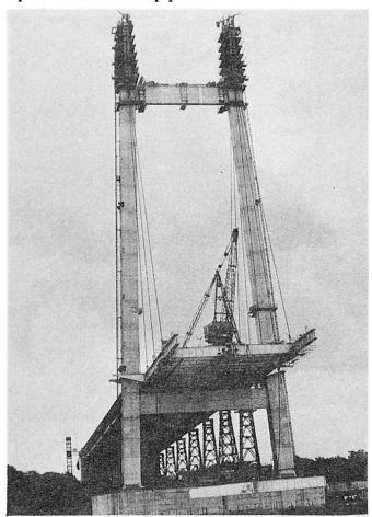
Fig. 1 H-shaped, 122 m high pylon at Calcutta side
