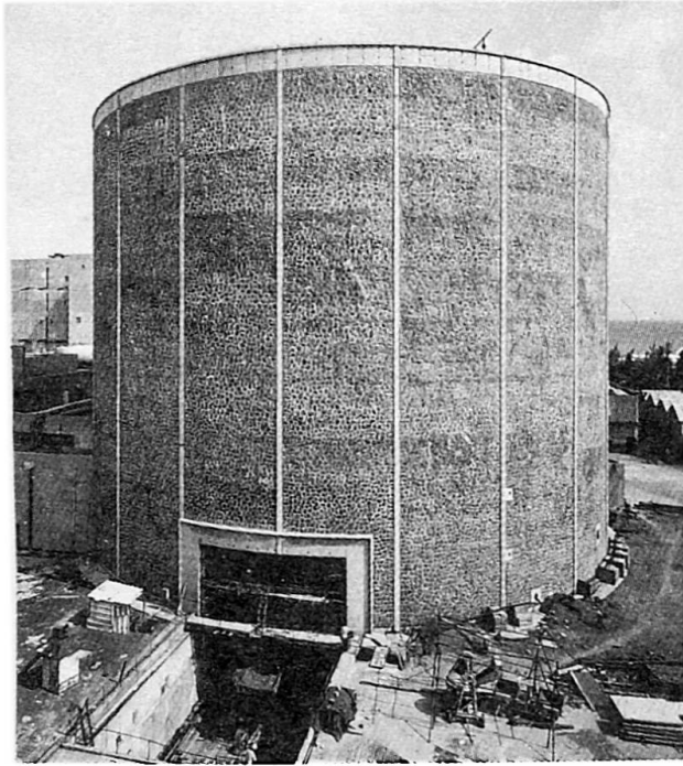
Fig.6 View of completed reactor, Madras
