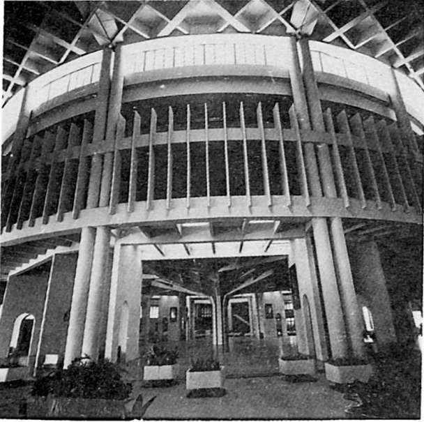
Fig.24 Assembly hall, Gandhinagar
