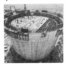
Fig. 2 Containment under Construction
