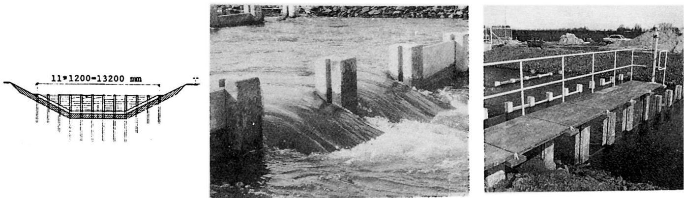
fig. 3: View of a weir fig. 4: piles and shutters fig. 5: foot-bridge
