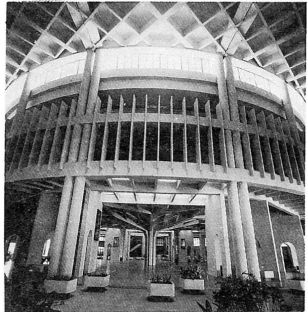
Fig.3 View of Assembly Hall from podium level
