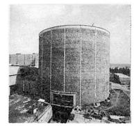
Fig. 4 MAPP - Masonry Wall & B.O.P. opening.
