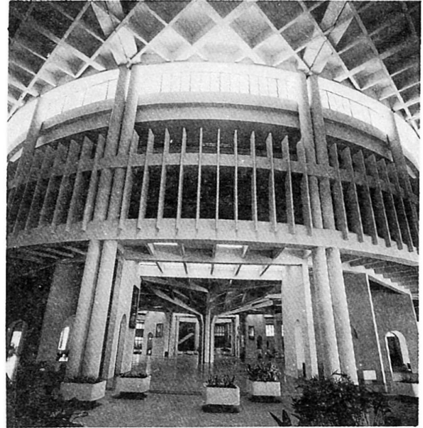
Fig.3 View of Assembly Hall from podium level
