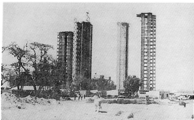
Fig.10 Slipformed Lift Cores
