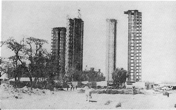
Fig.10 Slipformed Lift Cores
