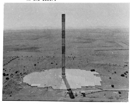
Fig. 2 Aerial photograph of the experimental facility at Manzanares, Spain (height of chimney 200 m; chimney radius 5 m; collector 120/120 m; rotor diameter 10 m; nominal speed 100 rpm)
