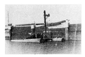
Photo.5 Launching camel placing RC planks
