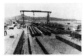
Photo.4 Casting yard for RC planks
