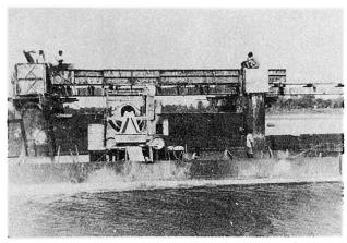
Photo 6 Concreting of cast in situ longitudingal bracings.
