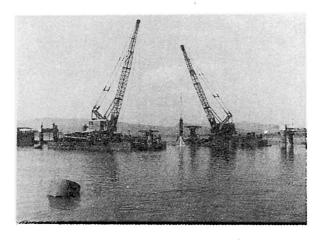
Photo.2 Hochstrasser piling rigs in operation
