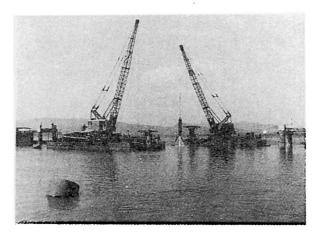
Photo.2 Hochstrasser piling rigs in operation
