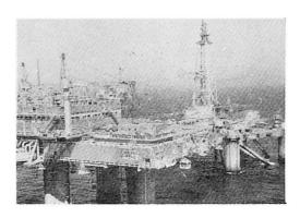
Fig. 2 Fixed gravity platform TCP2, Frigg North sea.
