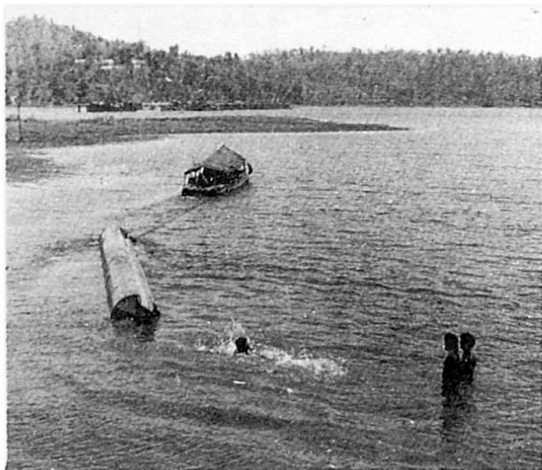
Photo.3 1000mm diameter casing being towed to site
