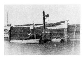
Photo.5 Launching camel placing RC planks
