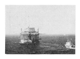
Fig. 4 Fixed gravity platform Doris, Frigg.
