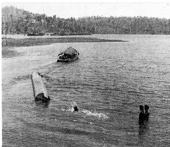
Photo.3 1000mm diameter casing being towed to site
