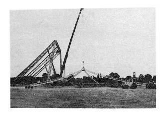
Figure 6 - Erection: raising pyramid
