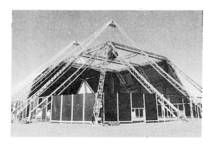
Figure 7 - Erection: installing fabric
