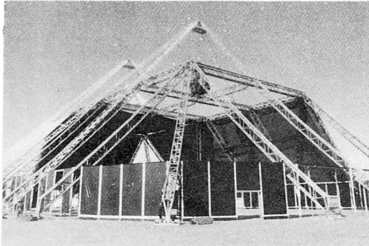
Figure 7 - Erection: installing fabric
